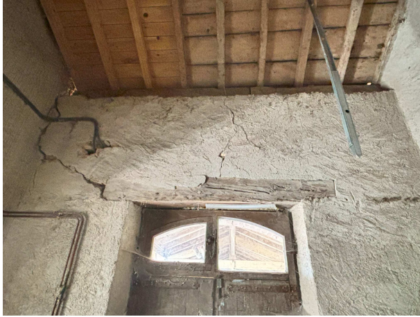
Figure 2 – Fissuration intérieure
