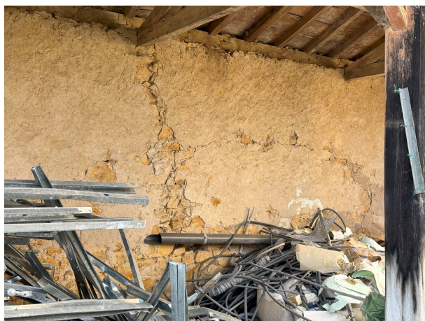
Figure 8 – Fissuration mur maçonné
